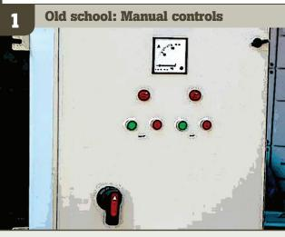
Plants that start, stop, and run manually almost always run at less than optimal production. The only real control an operator has after starting the plant is the speed of the feeders. Segregation occurs often within surge piles, creating fluctuations in material to crushers and constant gradation changes. To ensure that the plant doesn't have problems, the operator will run the feed at an "operator comfort zone" speed to handle the variables.
